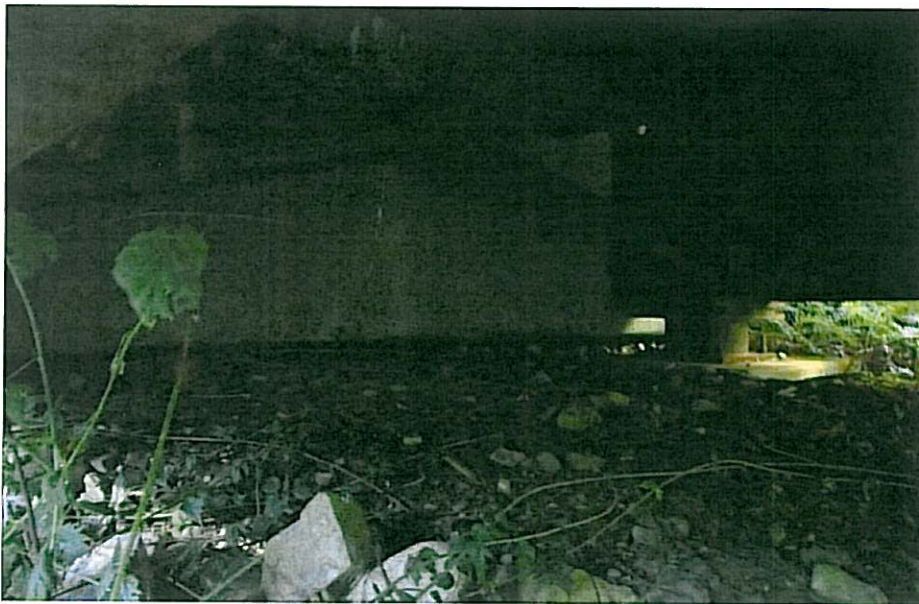
CK-2233 Right abutment
